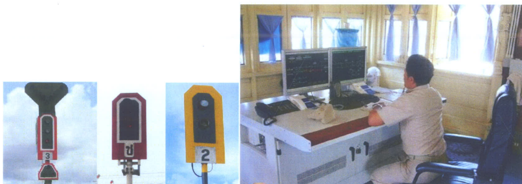
Figure 10.1-2 The Picture show Color Light Signals and Control Workstation at Station
