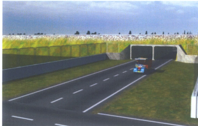
Figure 8-3 Box Culvert under Railway
