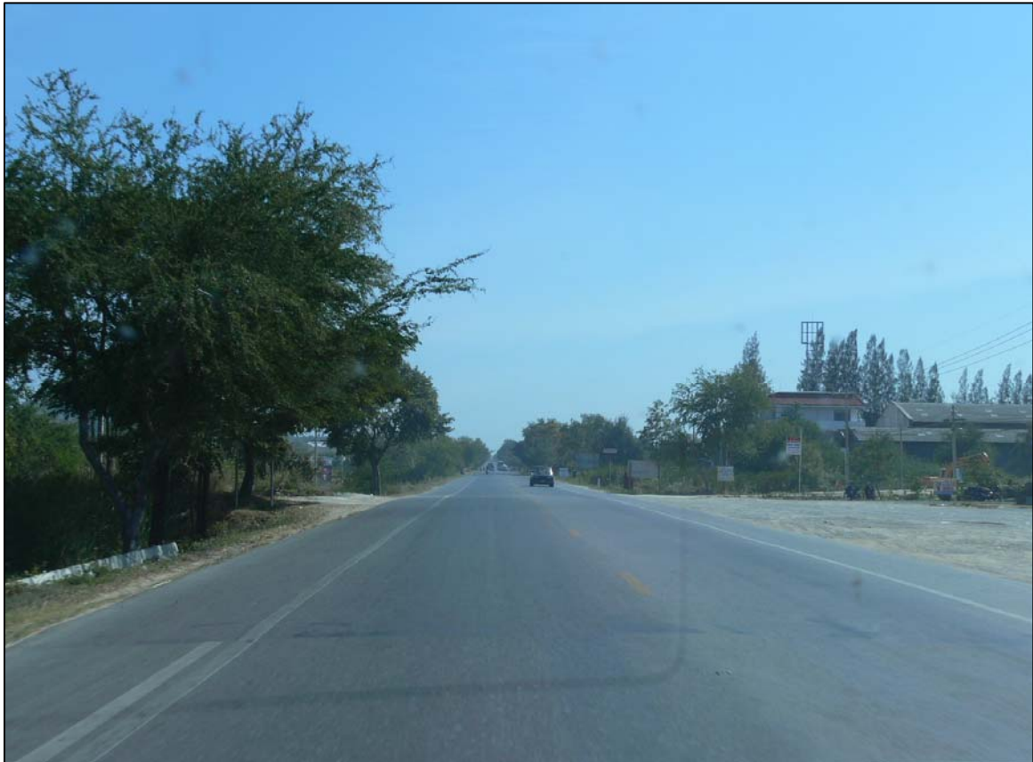
Figure 4.3-1(a) The current road condition A.HuaHin-Pranburi
