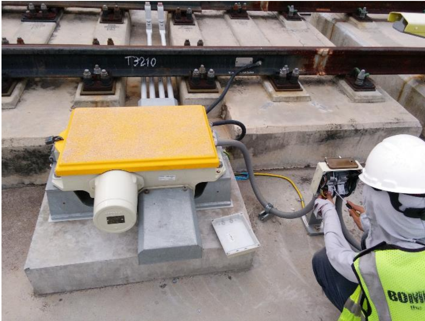
Signalling – Inspection of Point Machine and PLI before Testing
