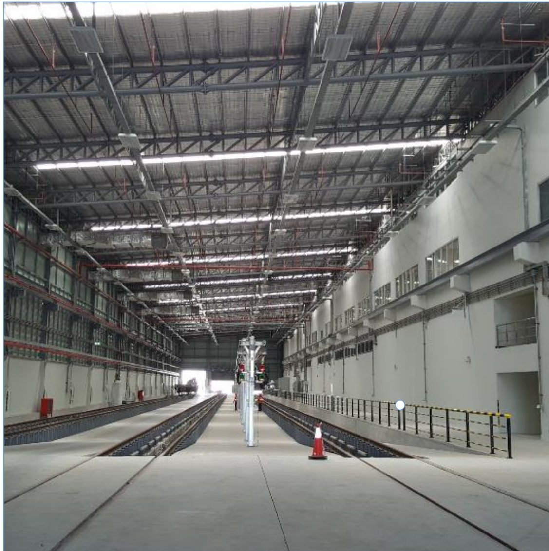
Power Supply – Stinger at Light Maintenance
