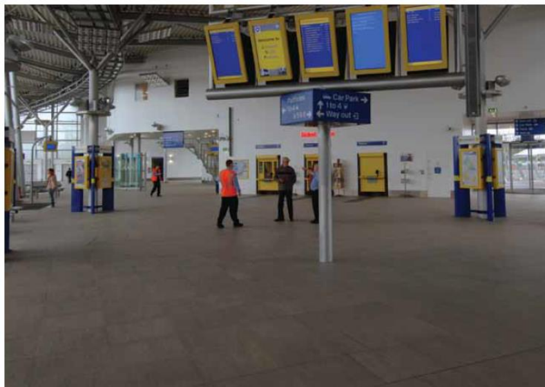
Figure I1.1 Station concourse with non-reflective floor
