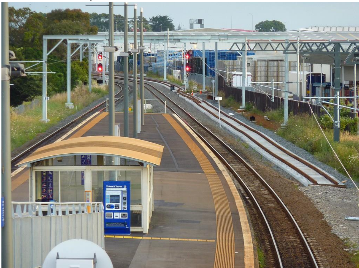
Puhinui Railway Station with ticket & top-up machine
