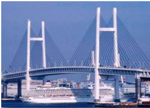
Structural Deterioration Analysis
